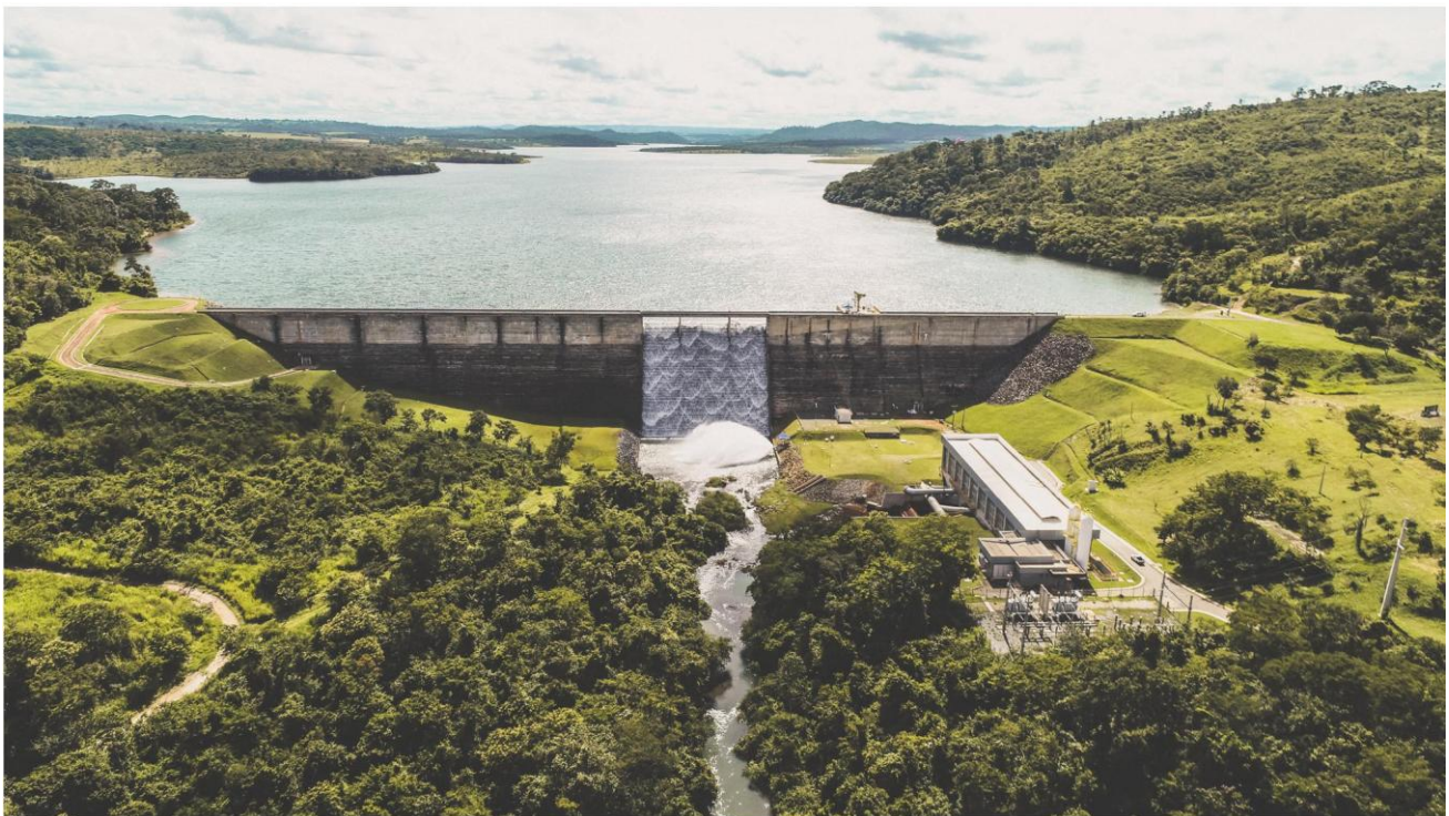
Figure 15 - Ribeirão João Leite Dam Source: Saneago
