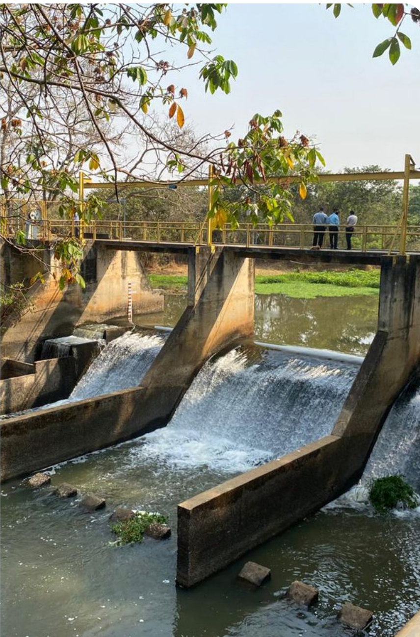
Meia Ponte River Dam / Saneago collection
