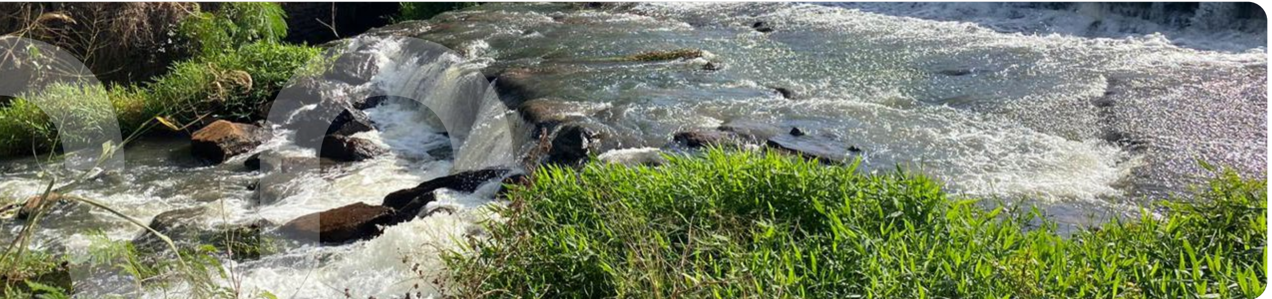
Água Branca Farm Dam
