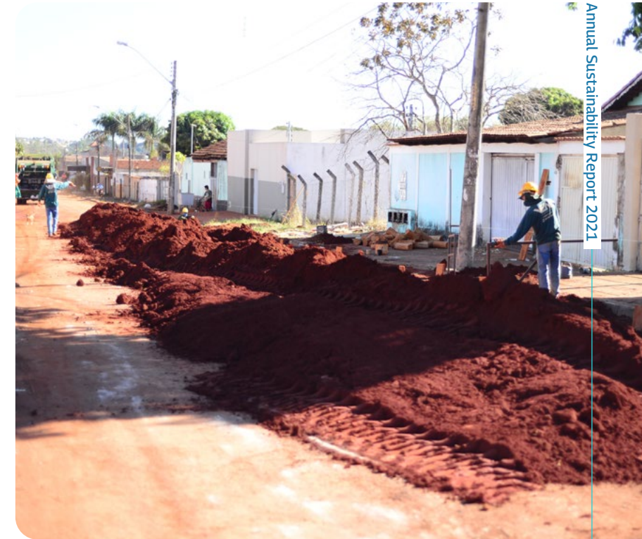
Expansion of the Goiânia's Sewage System
