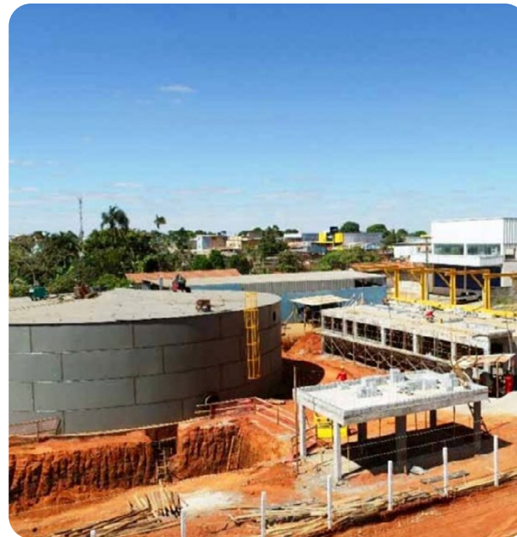
Expansion of the Aparecida Goiânia Water Supply System
