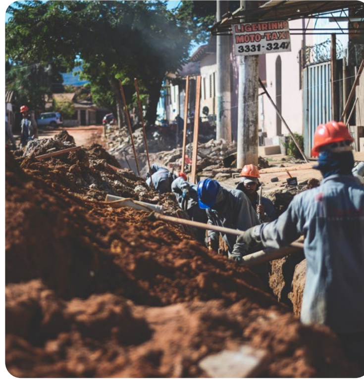
Expansion of the Pirenópolis Sewage System
