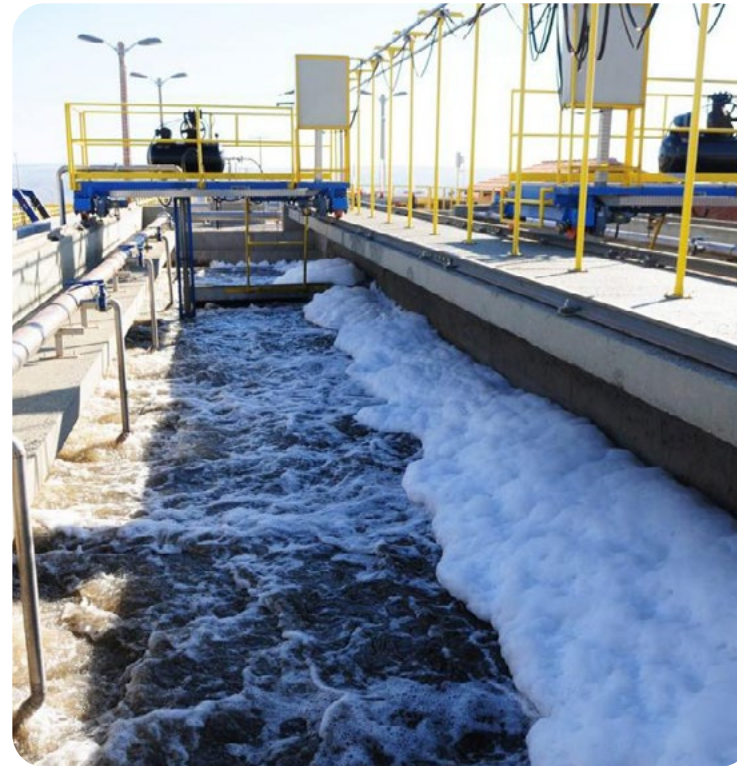
Corumbá WTP (Water Treatment Plant), in Valparaíso, GO
