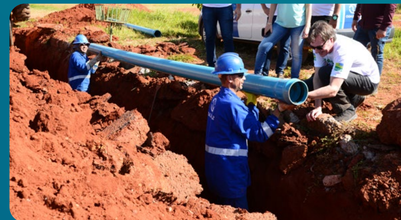
Building works in Valparaíso de Goiás - Saneago Collection
