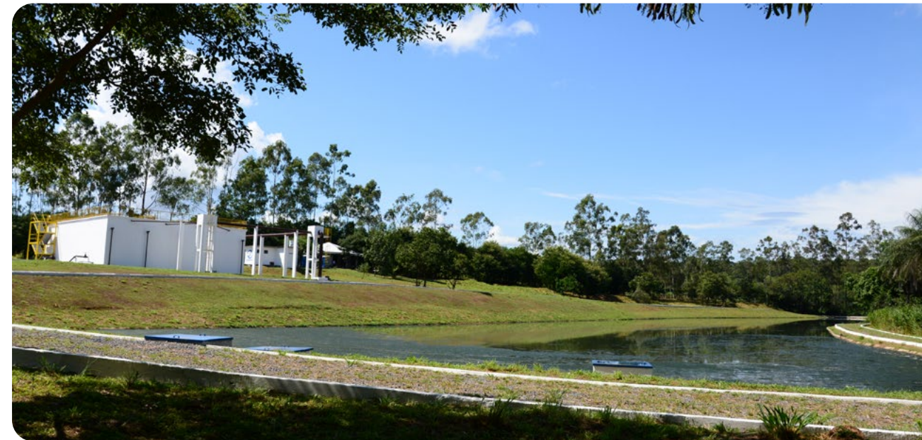
Posse Sewage Treatment Plant - Saneago Collection
