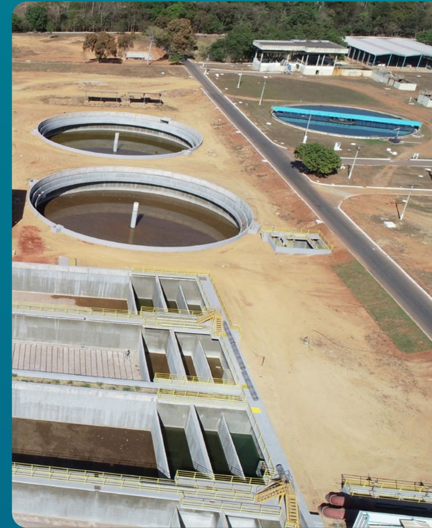
Goiânia Sewage Treatment Plant - Saneago Collection
