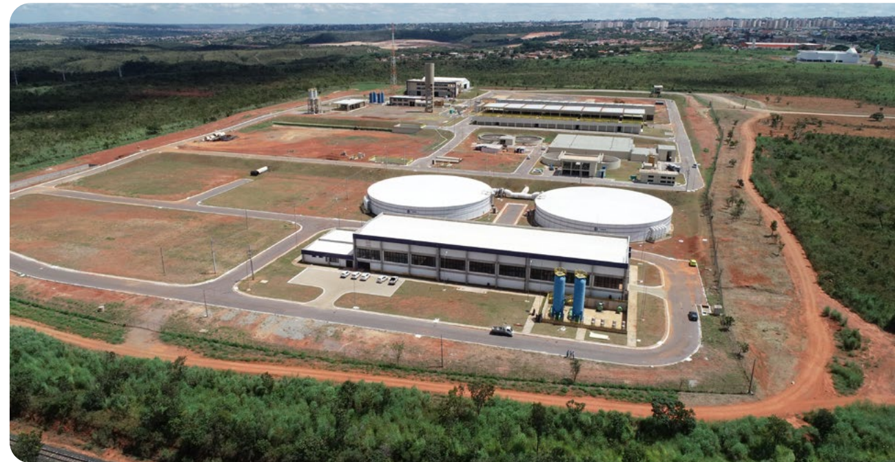
Corumbá System - Saneago Collection
